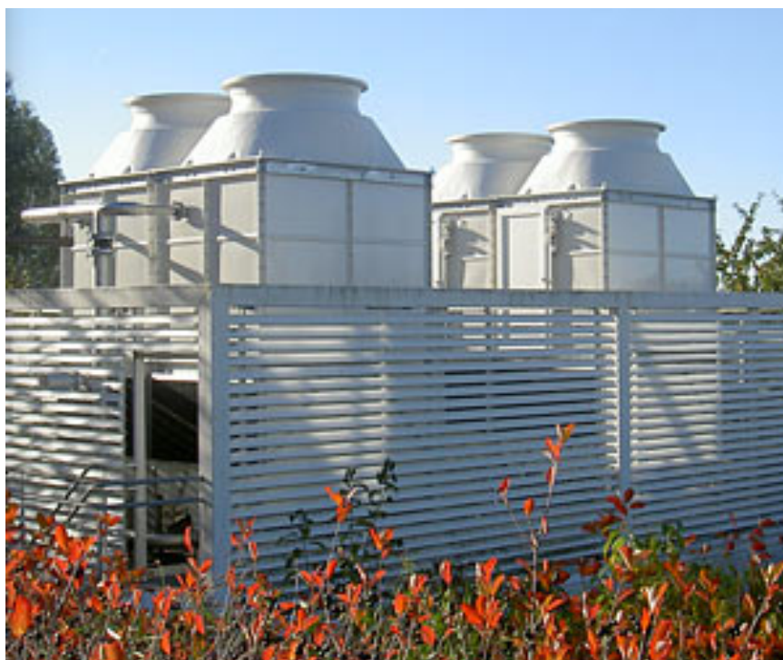
Figur 28. Modulkyltorn typ Vestas OCT05LHB02-2-120. SAS Flight Academy, Arlanda.
